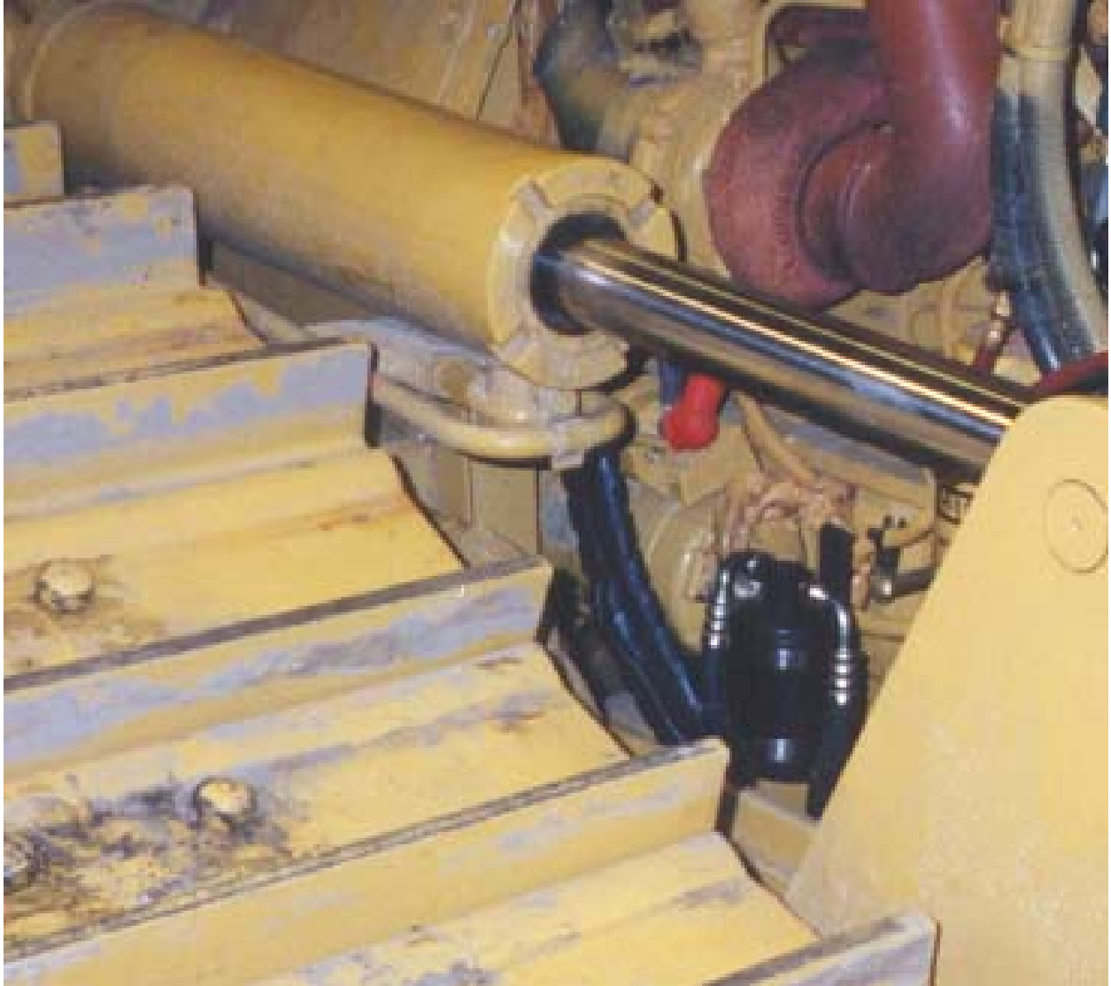
Drier location with hoses in place.
